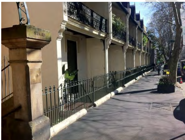
Photo 19: Victoria Street looking north from Butlers Stairs.
