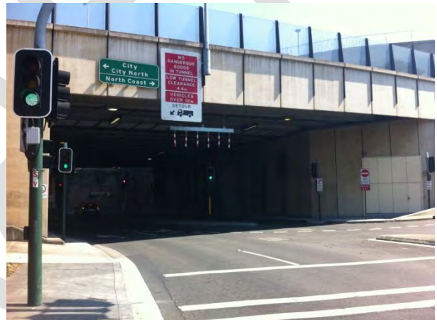
Photo 6: Cowper Wharf Road underpass below the Eastern Distributor
