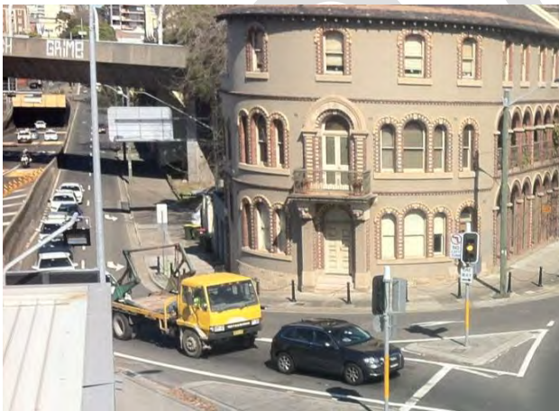
Photo 15: Palmer Street Low Point
