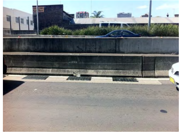
Photo 18: 4x0.6x1.0 m grated inlets
