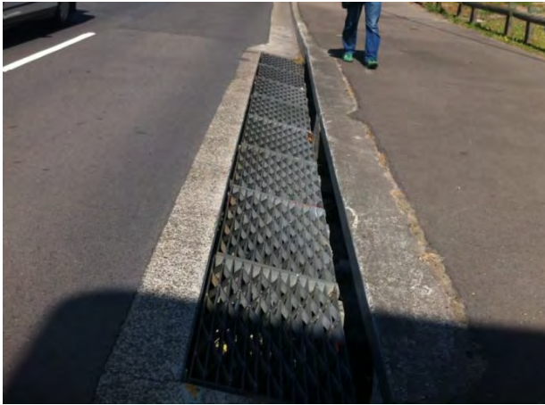
Photo 17: 7.2m lintel and 7x0.6x1.0 m grated inlets
