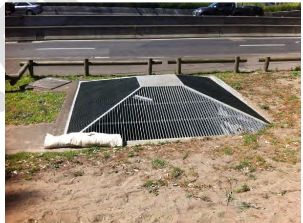
Photo 16: 4 m by 4 m inlet pit
