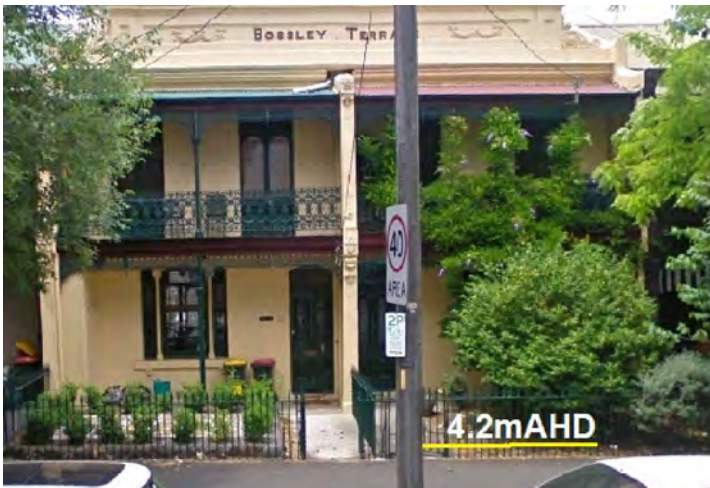
Approximate elevation of regular flooding along front fence near Crown Street Low Point.
